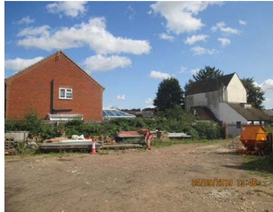
West elevation of no. 6 Meadow View
