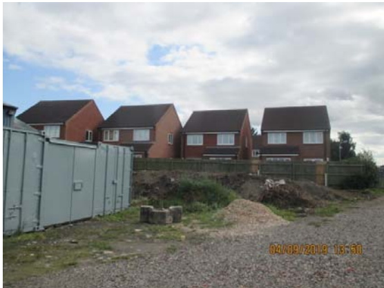
Rear elevation of nos. 6 – 9 Meadow View
